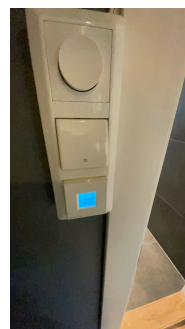
Termostatbryter for varmekabler.
