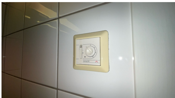
Termostatbryter for varmekabler.
