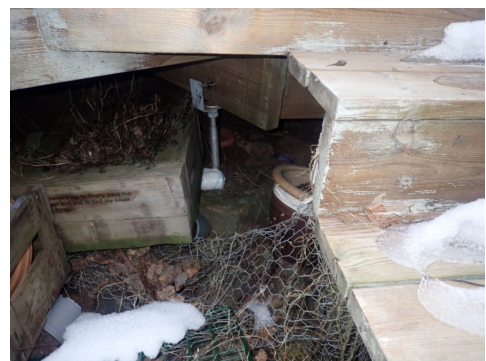
Fundament for terrasse
