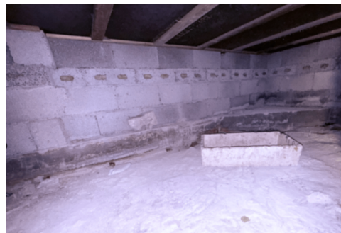
Mur i lettlinkerbetong.
